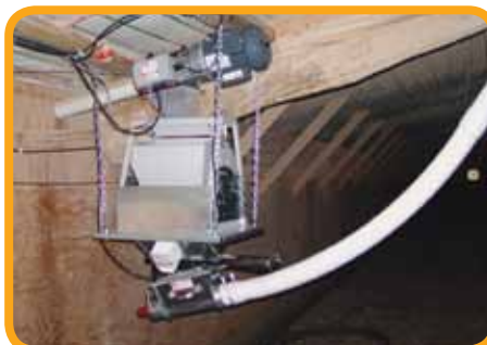
The CHORE-TIME® Feed Scale aids in scheduling feed deliveries and provides real-time data regarding feed inventory.
